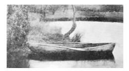
Figure 2. J. J. Lambot small reinforced concrete boat (1848).
